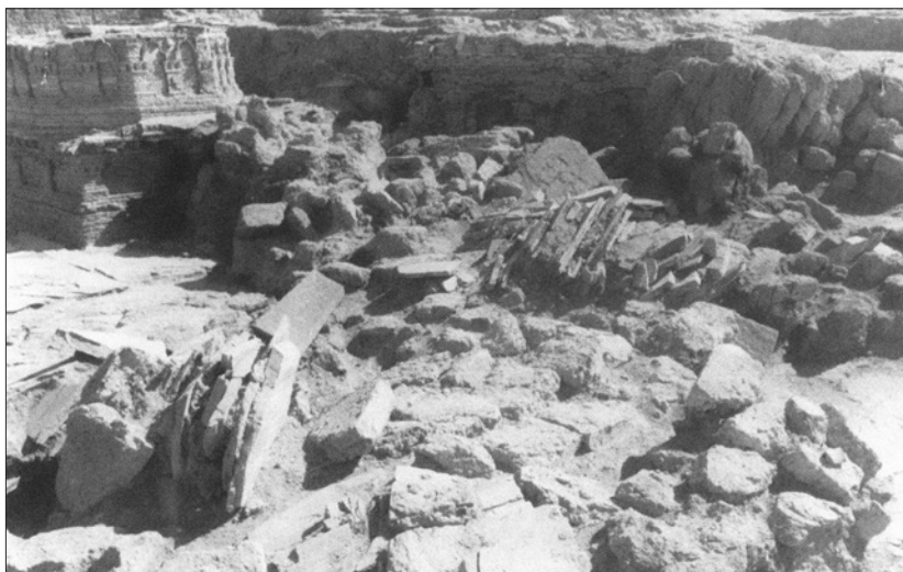
Figure 77. Collapses in the area of Stupa 64
